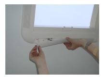
1.3.1 Install the HEKI 4 inner frame and connect the 12 Volt supply. Put the inner frame in place and fix with screws to the exterior frame using the smaller holes in the mounting block (screw 2,5x12)
